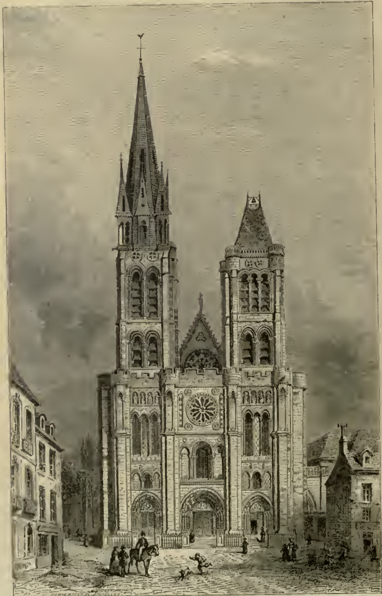
CATHEDRAL OF ST. DENIS; WITH NORTH TOWER BEFORE ITS DEMOLITION.
