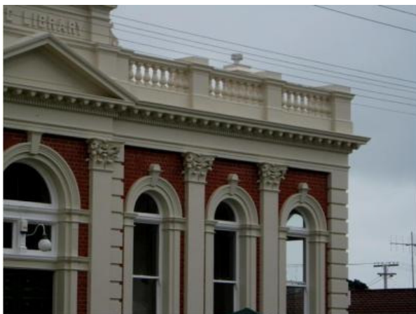
Restorations completed on Carnegie Free Library Building, Thames, New Zealand 2009
