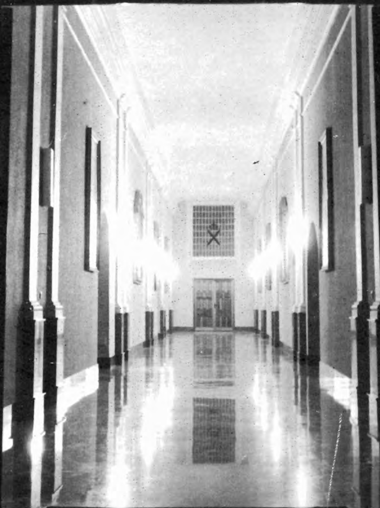
THE MAIN LOWER CORRIDOR (VALLADOLID)
