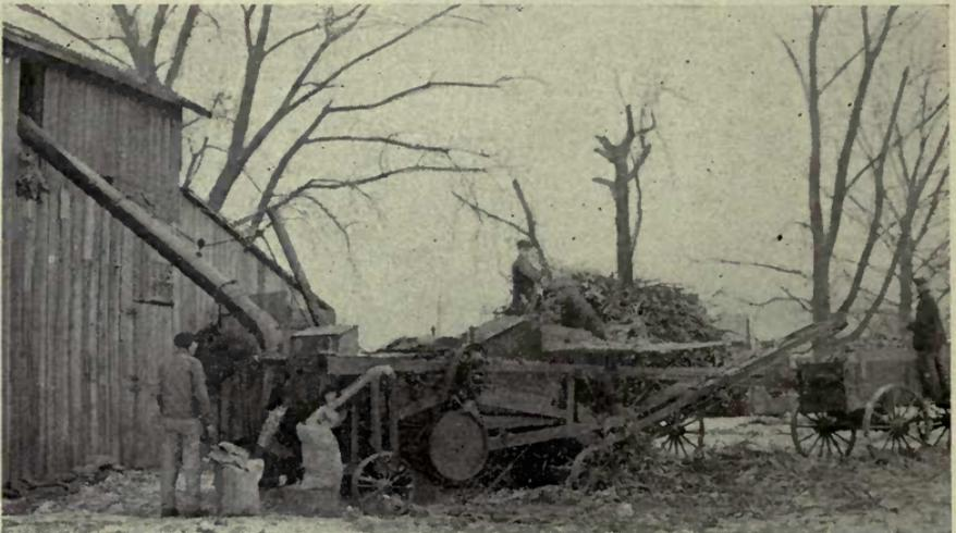
FIG 135.—The corn husker and shredder removes the ears and carries them to the rear where they may be caught in a wagon box. It shreds fodder very fine and blows it into a suitable storage place. Any corn shelled may be caught in bags, as shown. (I. H. Co.)
