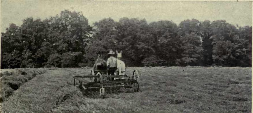
FIG. 109.—The side delivery hay rake rolls the hay into a wind row at one side. (I. H. Co.)
