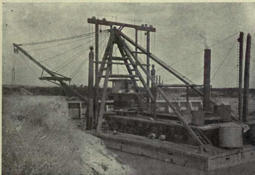
FIG. 89.—A dredge digging a ditch for irrigating an extensive area. (U. S. D. A.)
