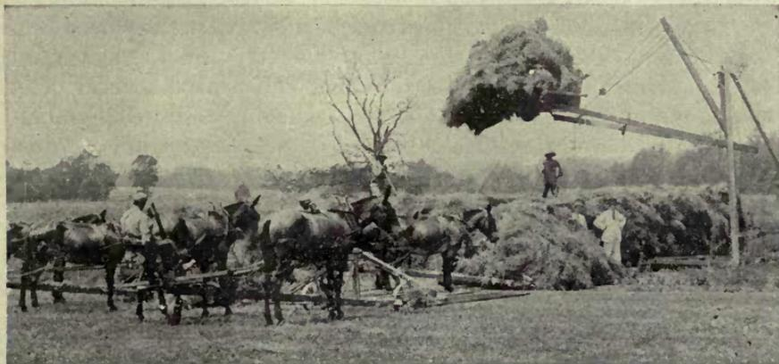
FIG. 123.—Stacking alfalfa in South Carolina. The hay is brought to the stack with rakes called "go-devils," and is then stacked with the crane stacker. (I. H. Co.)
