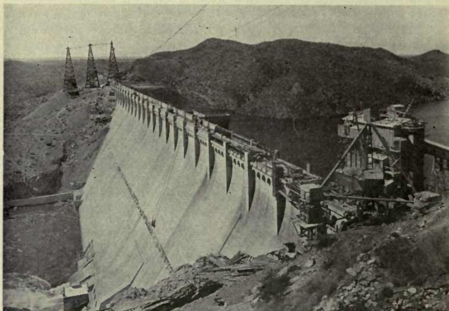
FIG. 88.—Elephant Butte dam, Messilla Valley, New Mexico, completed May 13, 1916. It is one of the largest re-enforced concrete dams of the United States Reclamation Service. In these projects the land is sold in small tracts to actual settlers only. (Courtesy Country Gentleman.)
