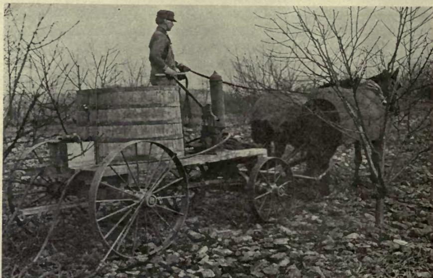
FIG. 293.▲—A spray pump operated by hand which pumps the liquid from the big tank and delivers it at high pressure through the spray hose. (New Jersey Station.)
