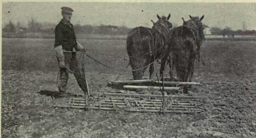
Fig. 74.—The common spike-tooth harrow is sometimes called a drag harrow. It is one of the best implements for smoothing the surface of the soil and producing a dust mulch to save the soil moisture. (New Jersey Station.)
