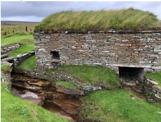
The water flows in, horizontally, on the opposite side of the building, at floor level, and falls through a vertical wheel (next photo), which is turned by the inertia of the flowing water, which then exits the building via the large opening on the right in the photo above.
