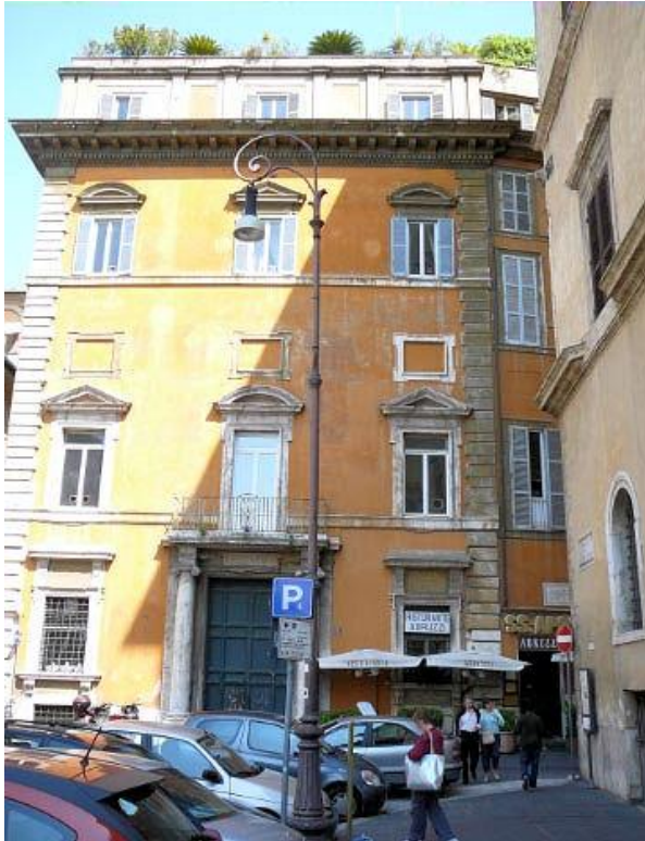
A portion of the front of Palazzo Muti
