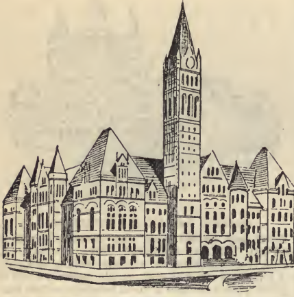
TORONTO MUNICIPAL BUILDINGS.
