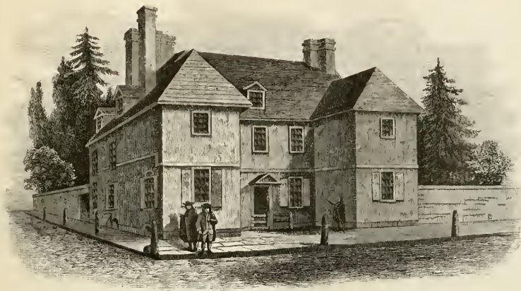
THE OLD SLATE-ROOF HOUSE.
