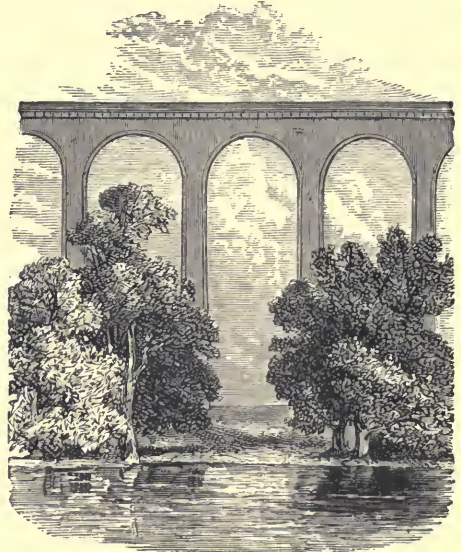
Middle Arches of the Dee Viaduct.
