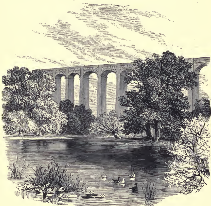
Aqueduct over the Dee.
