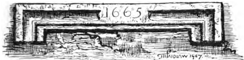
DOOR LINTEL, OLD HARWOOD HOUSE
