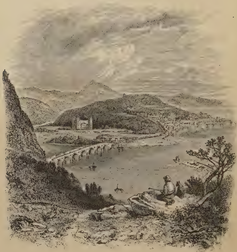
HANFF BRIDGE. [By R. P. Leitch ]
