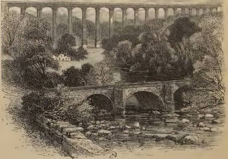
VIEW OF PONT-CYSYLLTAU AQUEDUCT.
