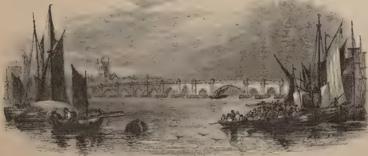
OLD LONDON BRIDGE AFTER THE REMOVAL OF THE HOUSES
