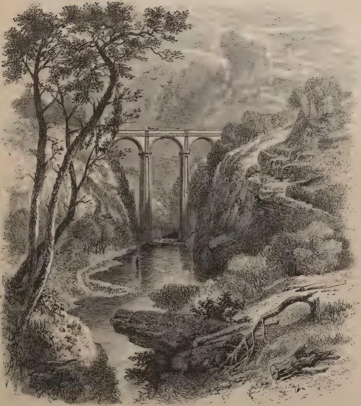
CARILAND CRAGS BRIDGE
