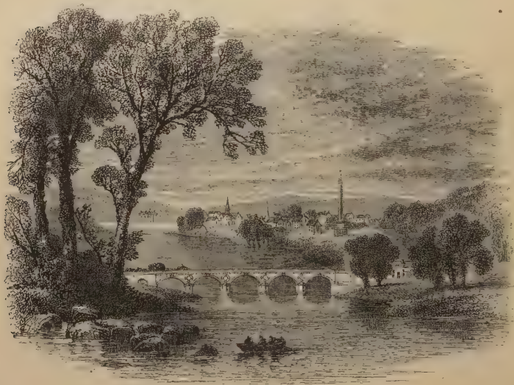
COLDSTREAM BRIDGE. [By E. M. Wimperis, after a drawing by J. S. Smiles.]
