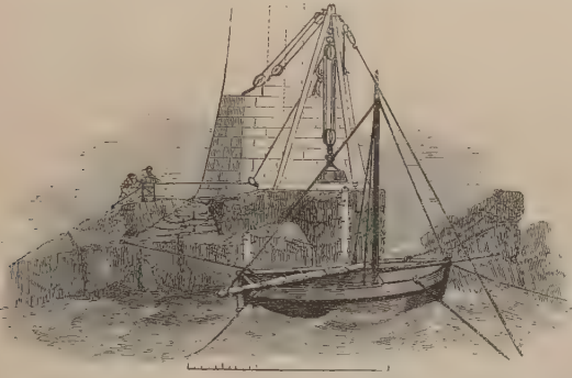
PROGRESS OF THE WORKS TO THE 16TH COURSE.
