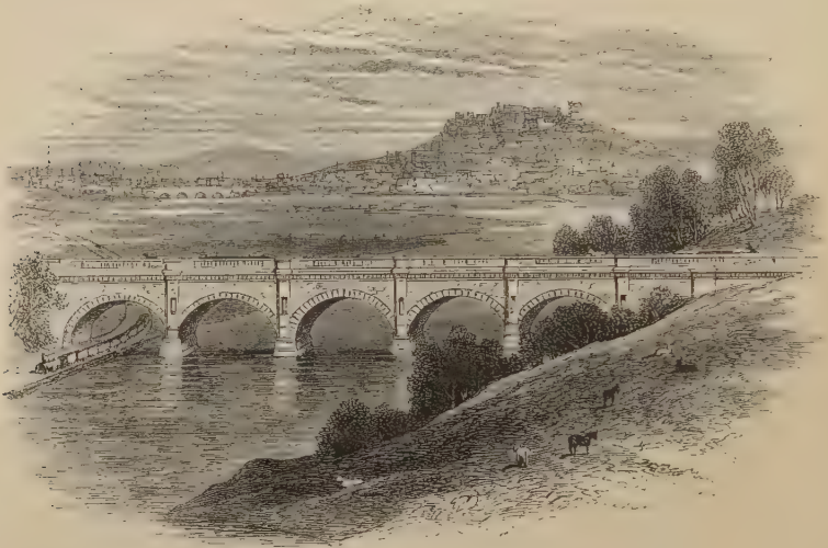
LUNE AQUEDUCT, NEAR LANCASTER.
