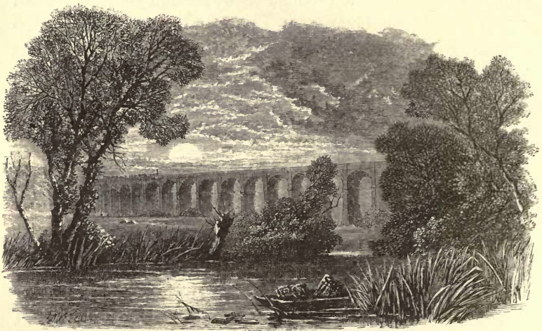
THE DUTTON VIADUCT.
