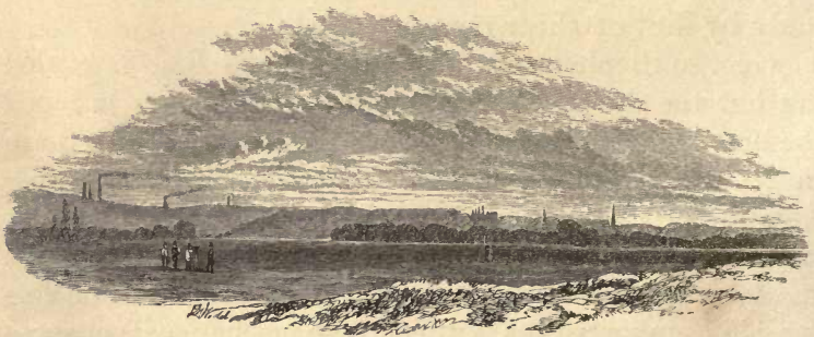
SURVEYING ON CHAT MOSS.
