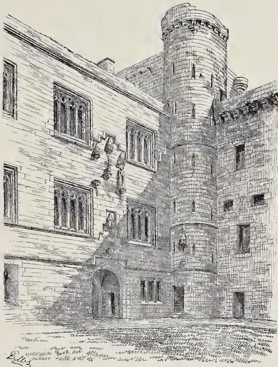
SOUTH-WEST ANGLE OF COURT OF LINLITHGOW PALACE.
