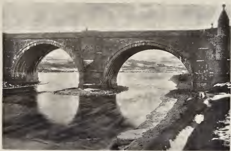
BRIDGE OVER THE DEE AT ABERDEEN.
