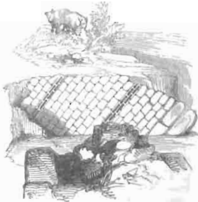
Postern entrance on the west.
