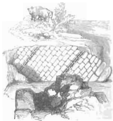
Postern entrance on the west.
