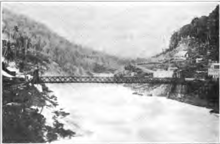
BRUNNERTON BRIDGE, OR THE GREY GORGE RAILWAY SUSPENSION BRIDGE.
