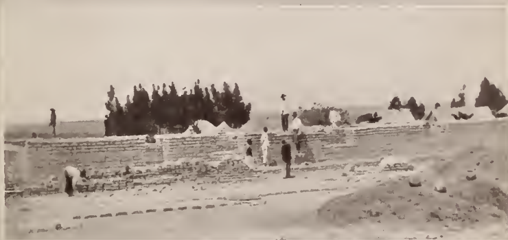
Sun dried mud brick building.
