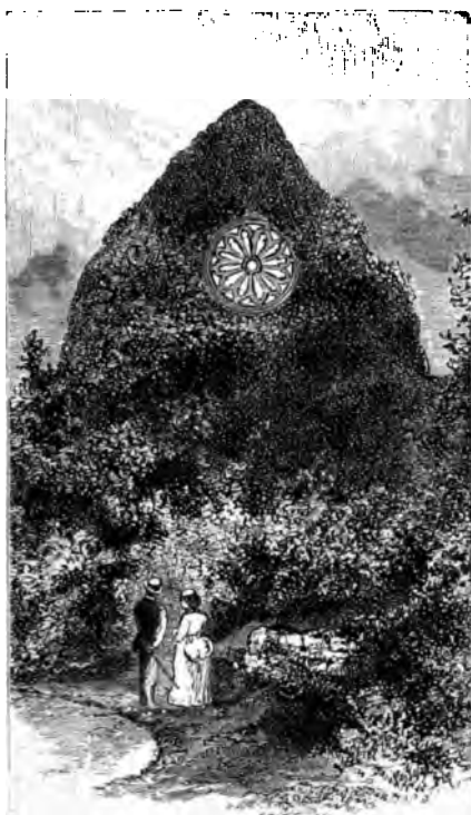
WINDOW IN THE REFECTORY.
