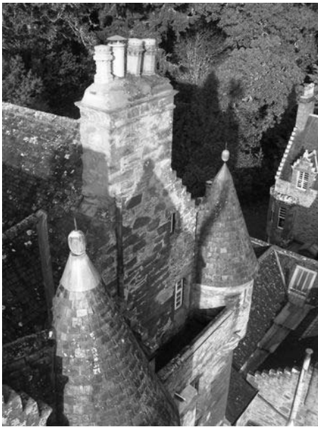
Castle Repair Work
