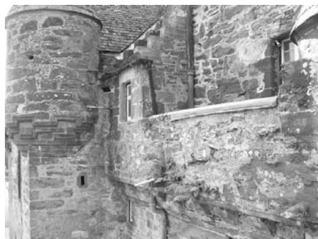
East Battlement before repairs
