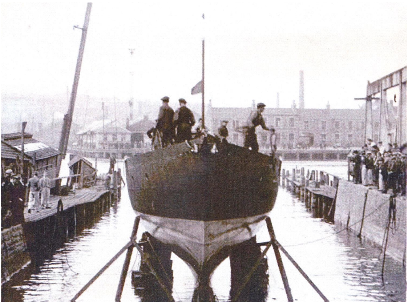
Launch of the yacht ‘Trenchemer’ using the Patent Slip. (Photographer unknown).
