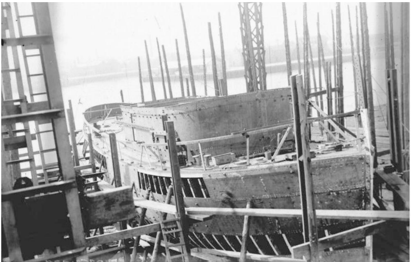
The hull of the 'Acklam Cross' under construction. (Hall Russell).
