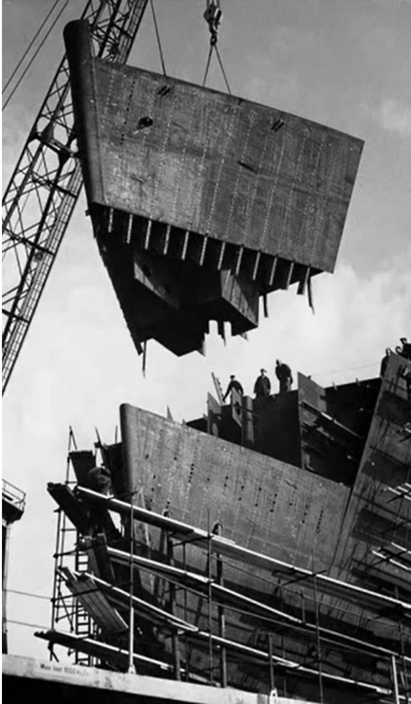
Erecting a bow unit c1960's. (Hall Russell).
