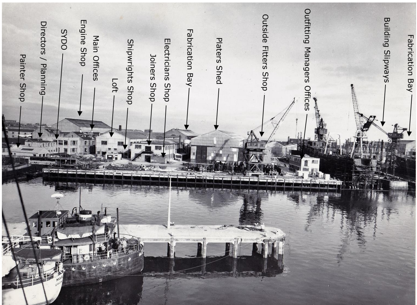
Hall Russell yard c1960. (Hall Russell). (Stern trawler on the slipway). (The 65-ton crane is not erected aside the Outfitting Managers block (right), however in this photograph you can see four large concrete blocks placed ready to take it.)
