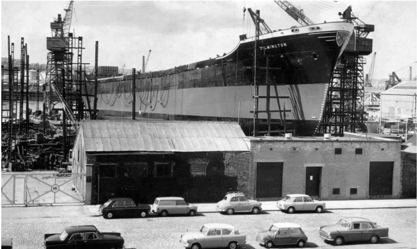
The bulk cargo vessel, 'Wilmington' pre-launch. (Hall Russell). (The shed next to the gate was the winch house for the Patent Slip).
