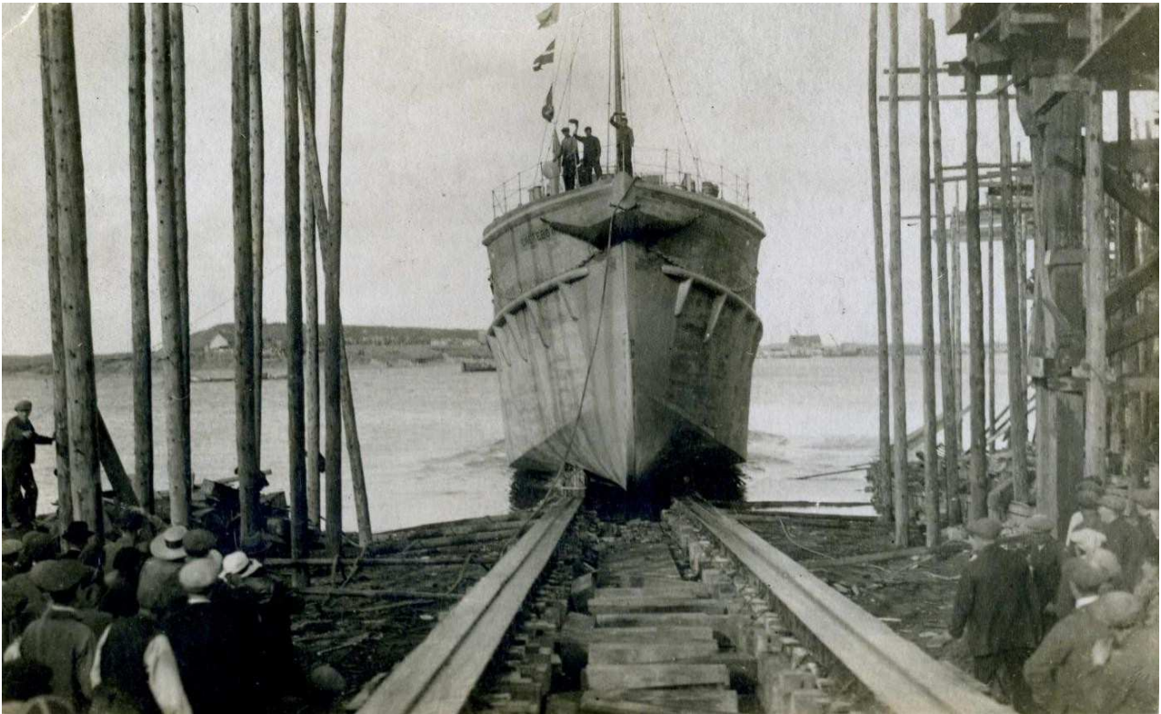
The concrete tug 'Cretebow'; being launched 31 st July 1919, at the Amble Ferro-Concrete Co. Ltd., The Braid, Amble, Northumberland. (Photographer unknown).
