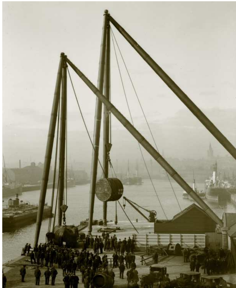
Load test of the new 100 ton Sheer Legs, 3 rd September 1910. (3 days before the launch of the SS 'Intaba'). (Photographer unknown).
