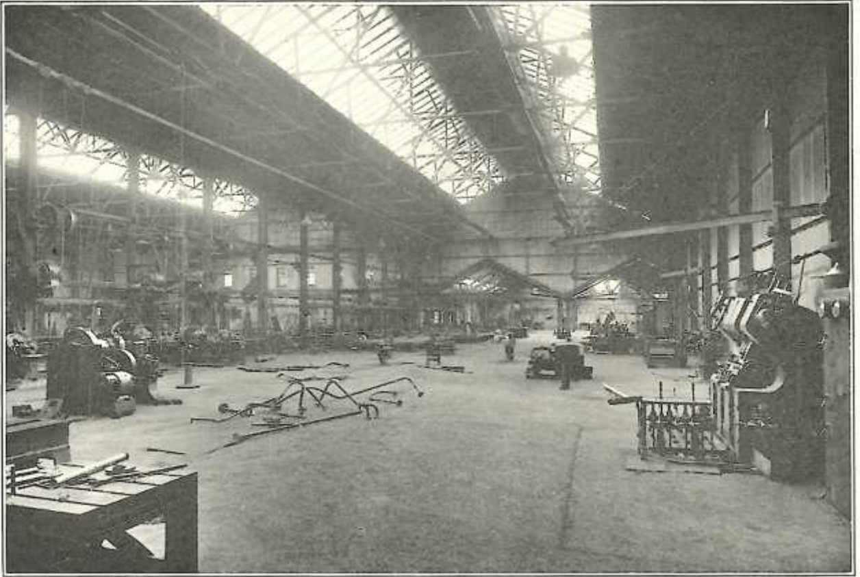
New Plumbers' Shop.
