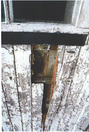
13. The sawn log construction is clearly visible where the siding has been broken. The strapping is old wood indicating that the logs may have had siding added at an early date.
