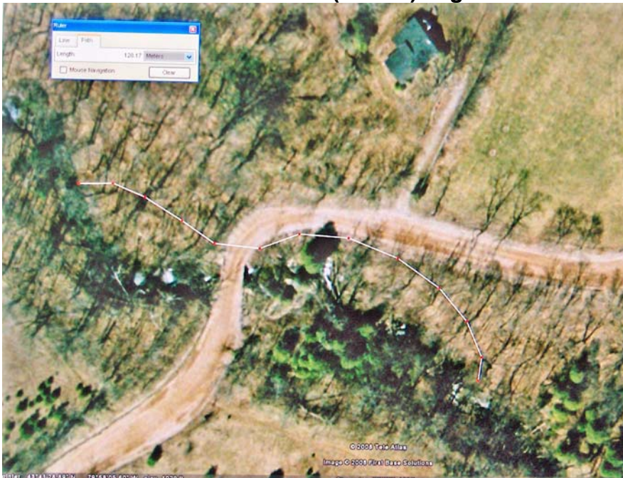
4.27 Aerial Photo of the probable (130 m.) alignment of sluice boxes for the lower mill. The additional 20 metres of sluice would bring the same volume of water from almost 10 feet (3 metres) higher.
