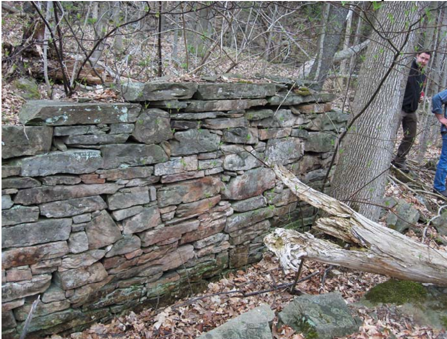
4.17 Portion of earth embanked wall which supported bearing blocks for millwheel. Large (20") hardwood tree has grown up on the debris and stone which has filled the trench. Rob Kier (black jacket in background) a resident of the house, found these walls in 1961.
