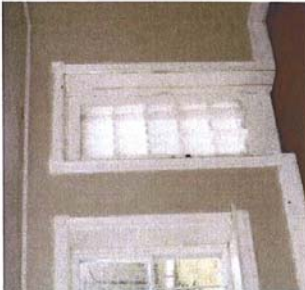
25. Detail showing thick walls at front door and window.
