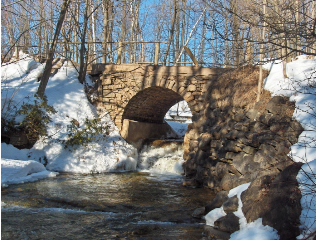
5/06 Silver Creek Bridge (sandstone bedded in lime mortar, single vault) Note modern concrete abutments added to reinforce base of arch, and wooden railing installed on concrete cap laid over masonry. © T.Murison 2008
