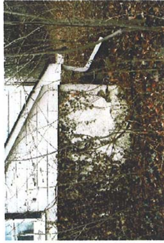
8. Close up of the utility/cold cellar wall. Plaster on stone.
