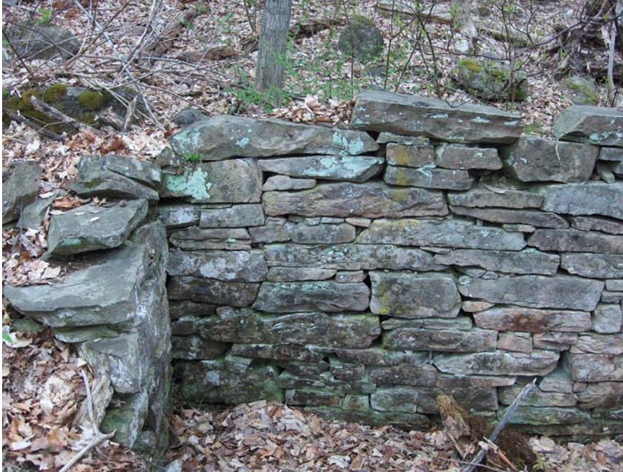
4.16 N.E. corner of stone foundation for mill wheel. Upstream end wall at left.
