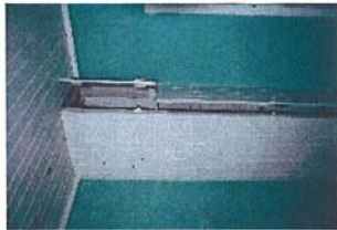
24. Closet in S-W bedroom.
