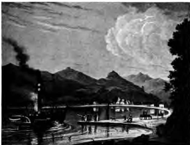
AT LOCH GOIL JETTY
