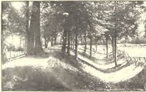
EMBANKMENT WITH INTERIOR MOAT, NEWARK WORKS
