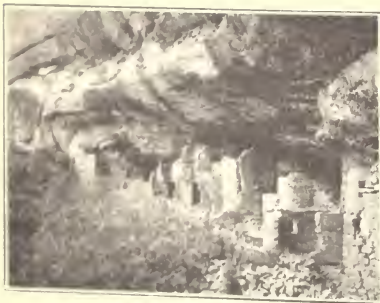
SPRUCETREE HOUSE, BEFORE REPAIR
