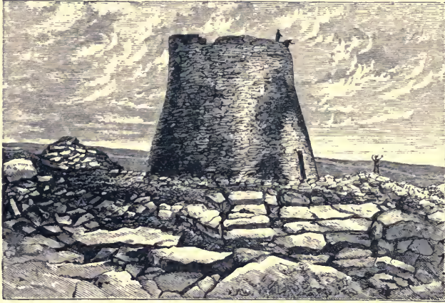
Fig. 160.—Exterior View of the Broch of Mousa, Shetland.
