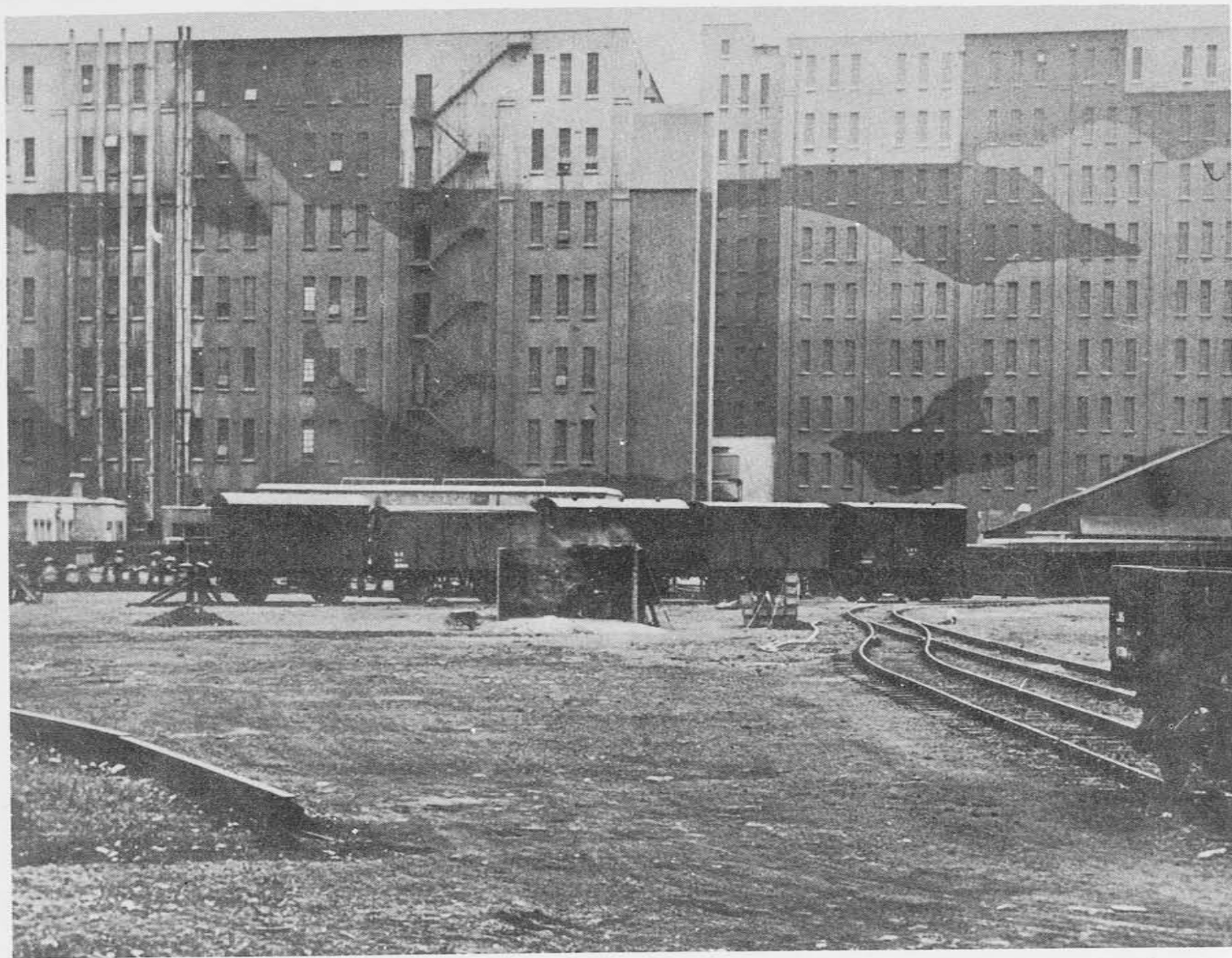
FIGURE 11.—A Warehouse at Bristol.
