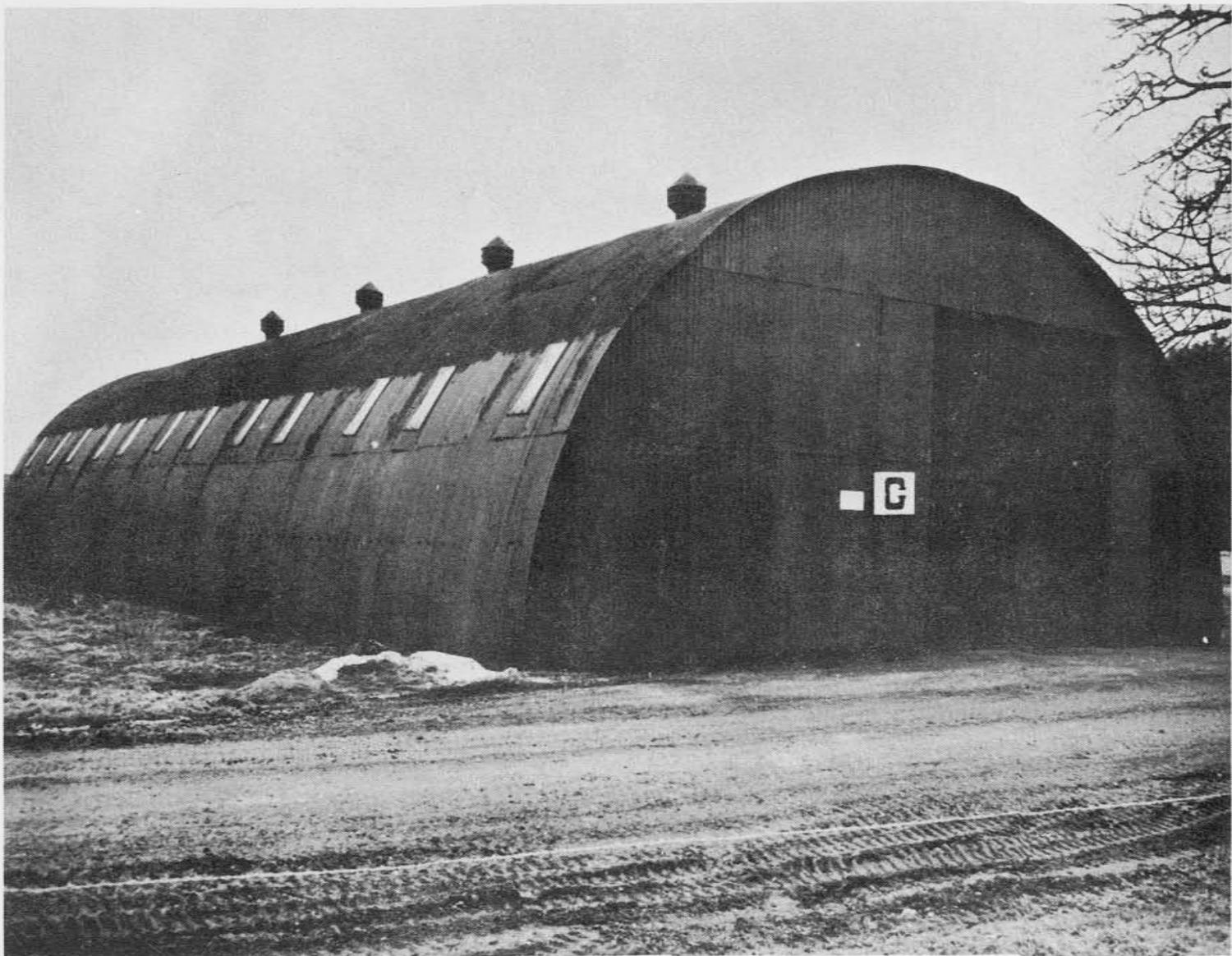
FIGURE 2.—Nissen Hut Completed for Salvage Storage.
