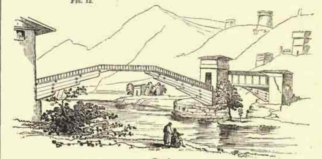
FIG. 9. TYPES OF CANTILEVER BRIDGES.
