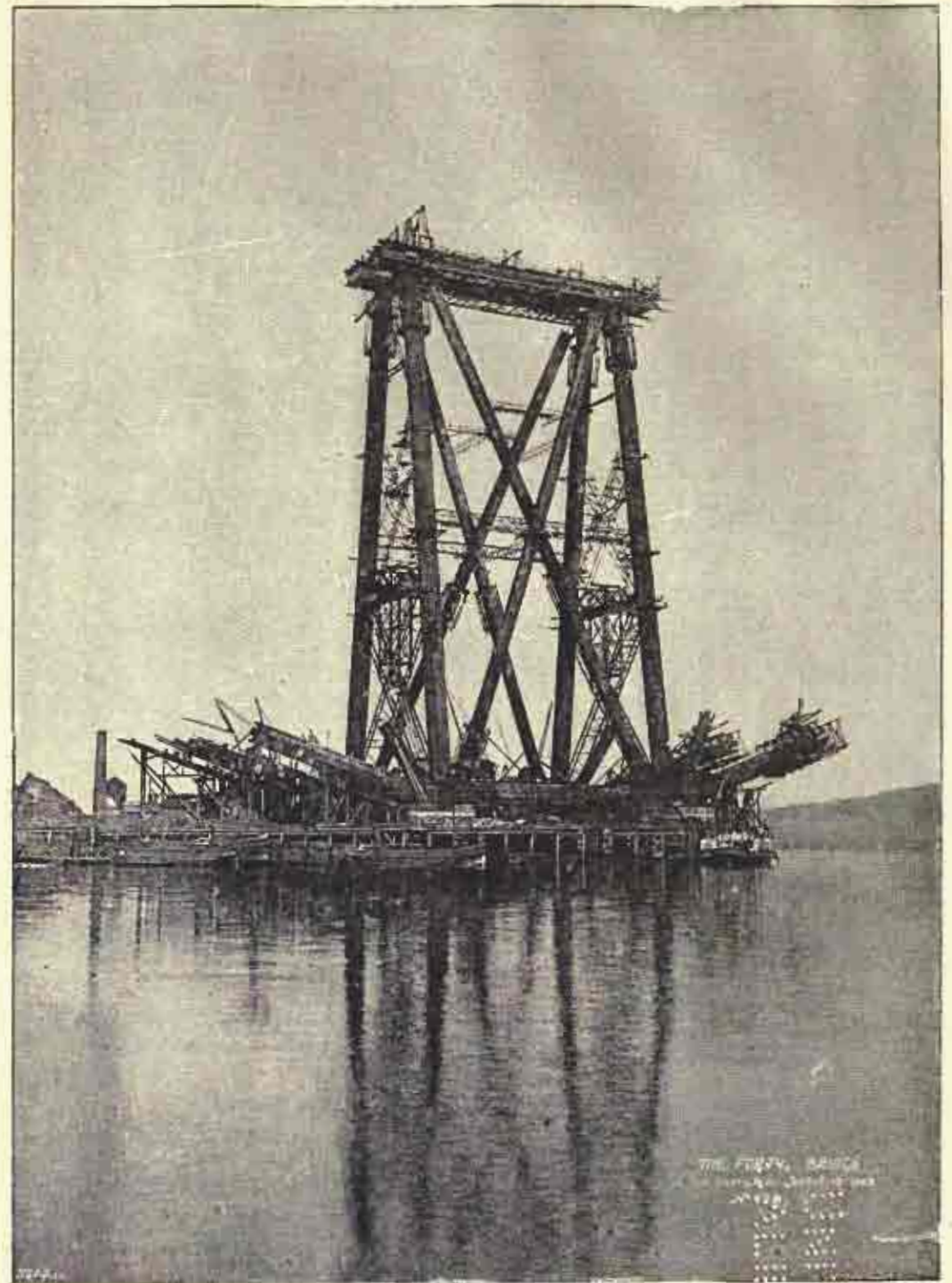
PIE PIER. PLATFORMS RAISED TO FULL HEIGHT.
