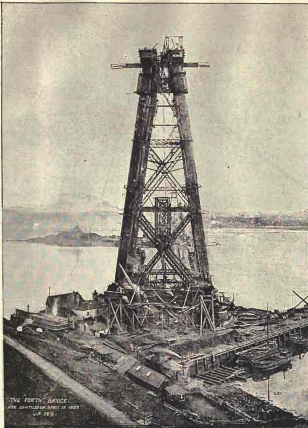
PIE PIER, LOOKING SOUTH. PLATFORMS RAISED TO FULL HEIGHT.
