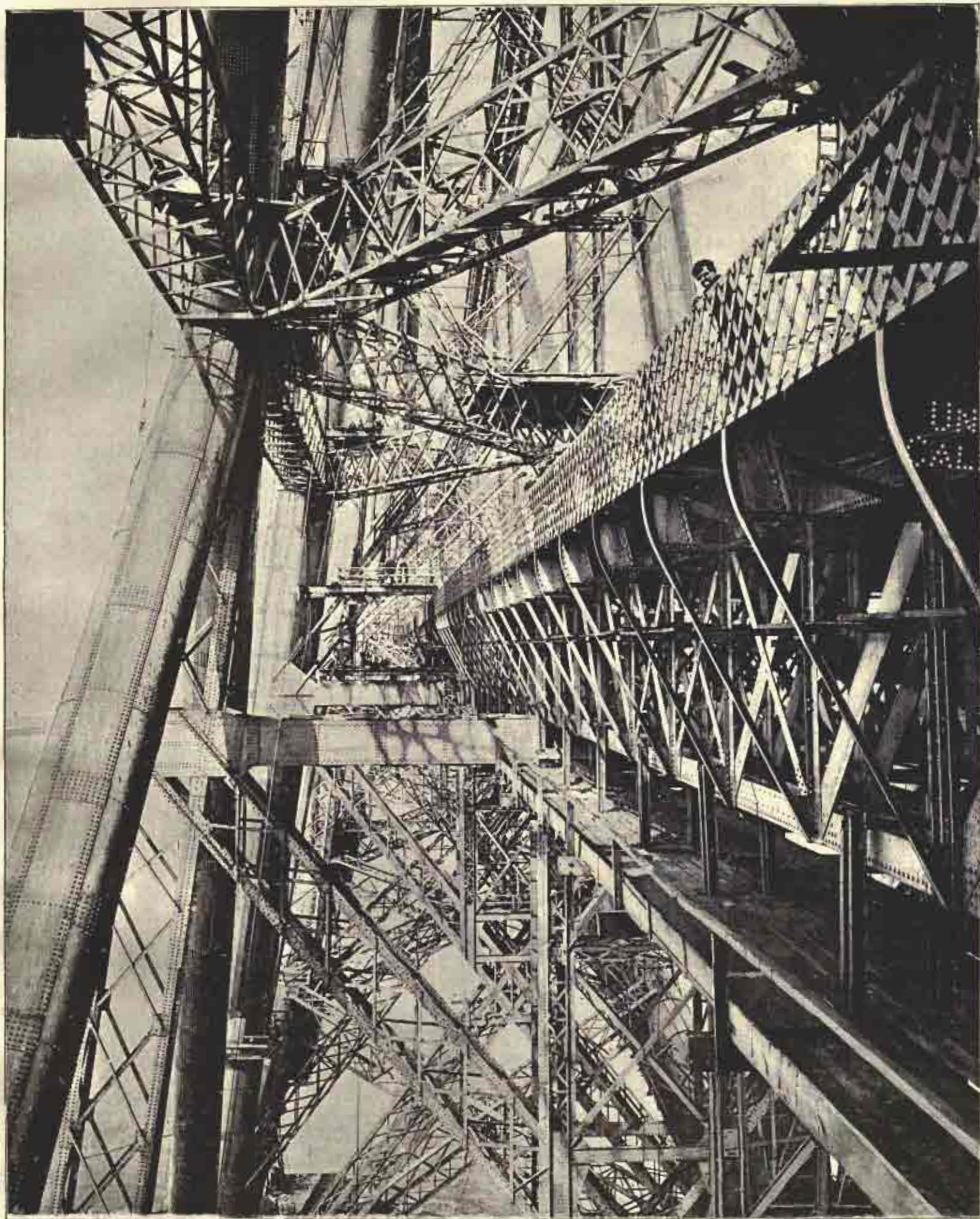
CENTRAL TOWER OF INCHGARVIE; INTERNAL VIADUCT GIRDERS AND WIND FENCE.
