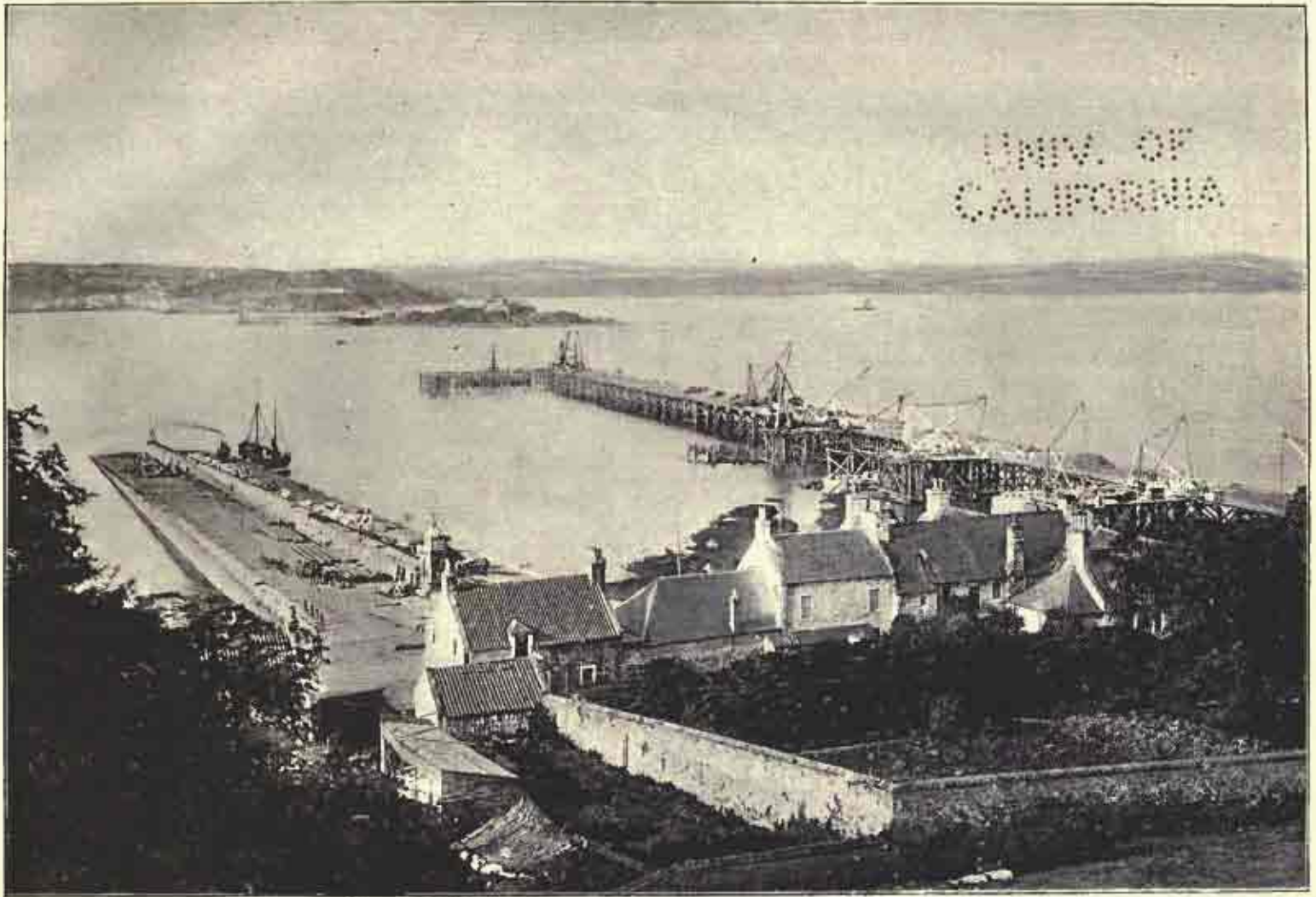
GENERAL VIEW OF SITE LOOKING NORTH-EAST.
