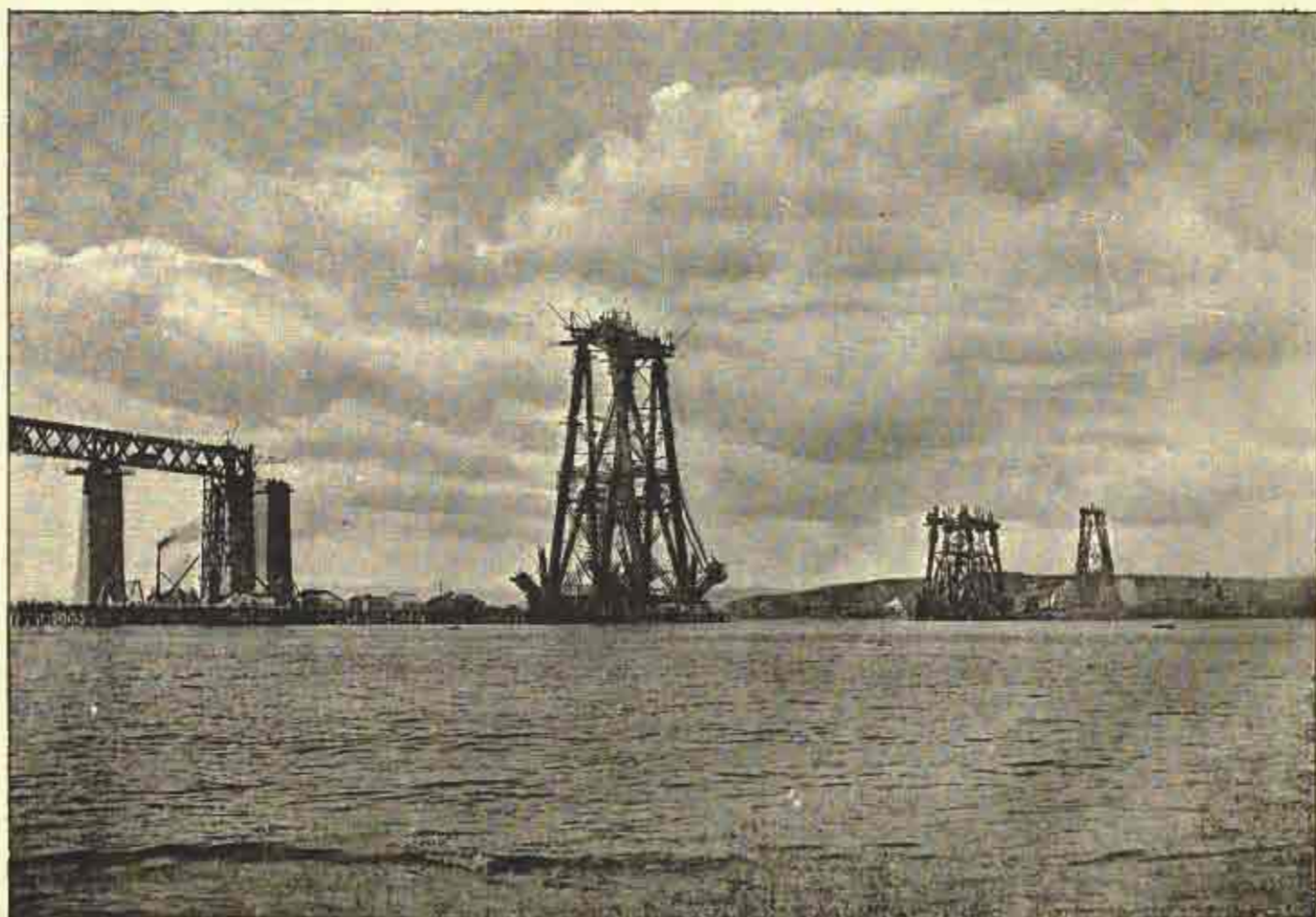
GENERAL VIEW OF CENTRAL TOWERS AND APPROACH VIADUCTS LOOKING NORTH.
