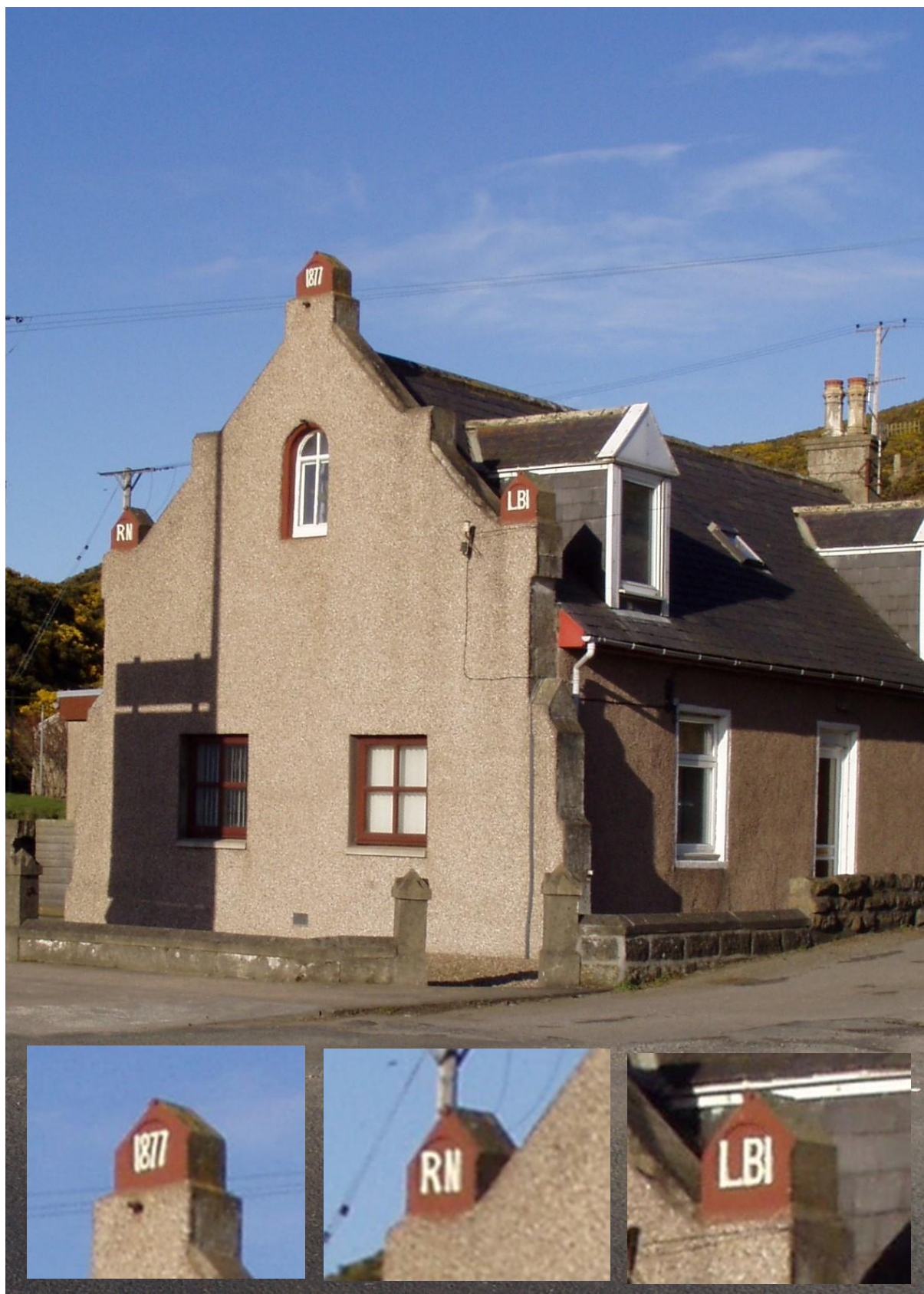
Former Lifeboat House at east side of Banff Bridge, 'RN LBI 1877'. (S. Bruce).
