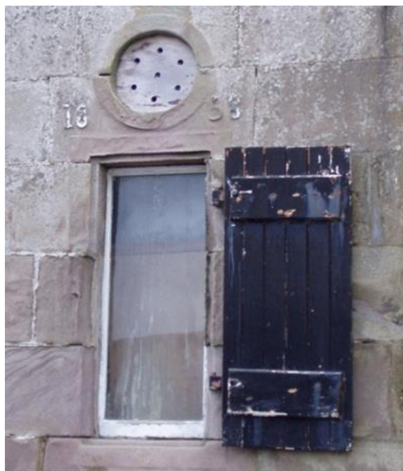
Whitehills former barometer box of 1858, No. 37 Low Shore, Whitehills. (S. Bruce).
