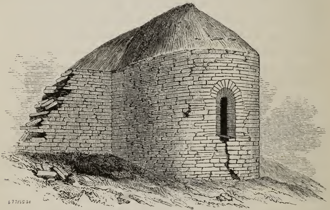
FIG. 187.—Girth House of Orphir.
