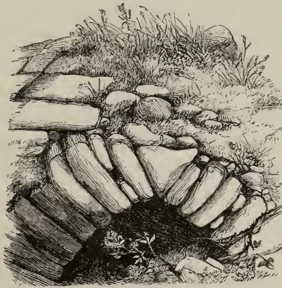
FIG. 189.— Vaulted Ceiling, Inchcolm.
