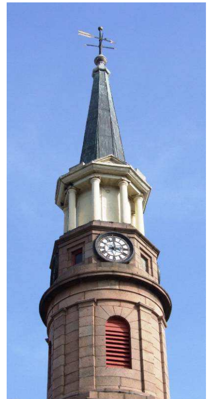
The County building (1826) 130' high clock and spire (1856/57).
