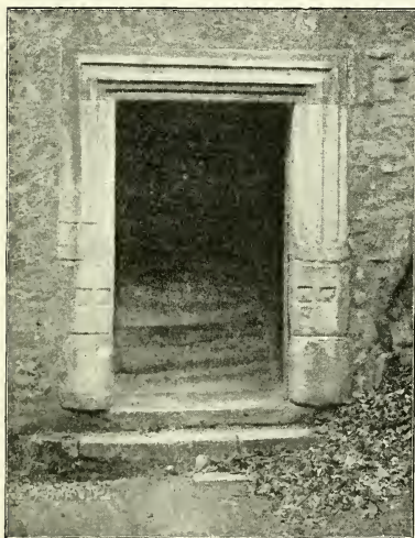
DOORWAY TO MAIN STAIRCASE.
