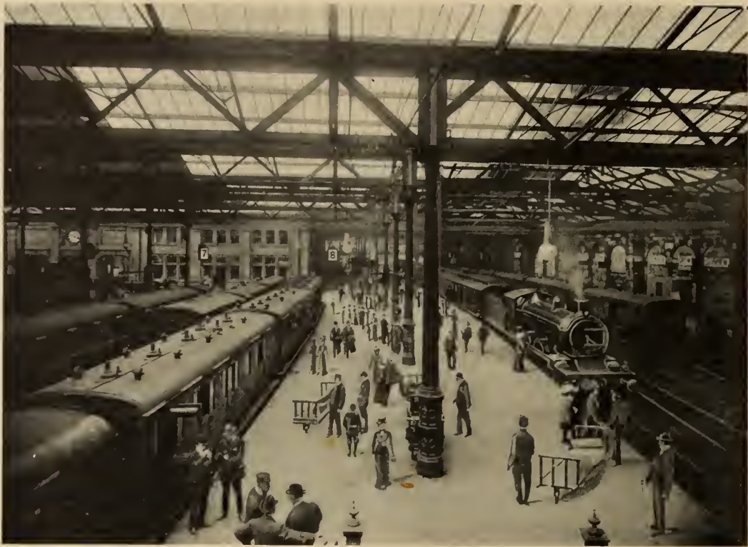
UP MAIN PLATFORM (EAST END), WAVERLEY STATION
