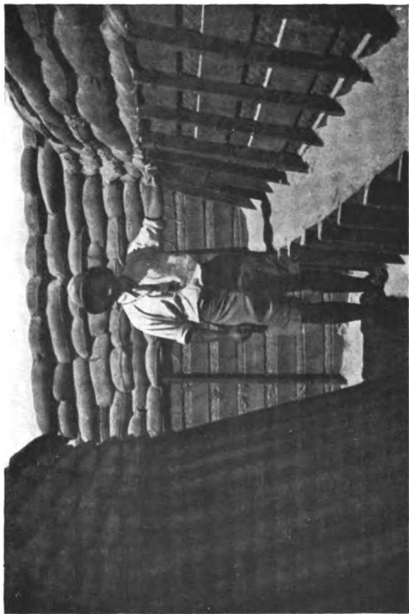
IN NO. 4 POST, ROMANI, SHOWING COMMON TYPE OF TRENCH IN REDOUBT
