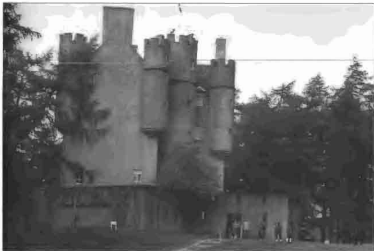
Braemar Castle, a typical example of an "L Plan" tower house forming a chief's residence. The Jacobite standard was raised outside in 1715. [Author's collection]
