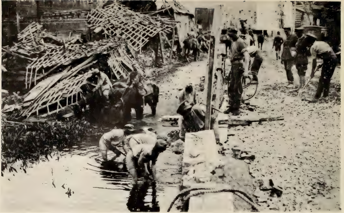
CANADIAN ENGINEERS FILLING IN THE CRATER BLOWN BY THE GERMANS IN THE BRIDGE AT HANGARD.
