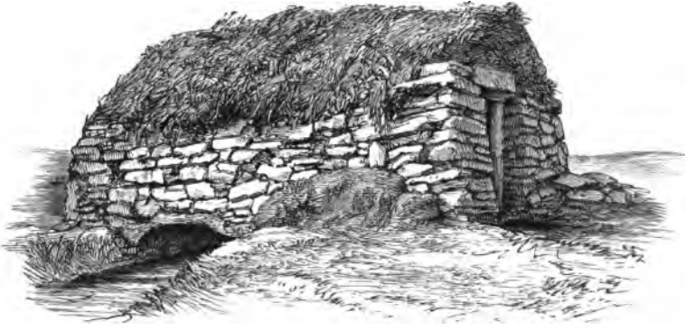
Mill at Sound, near Lerwick (from a photograph).
