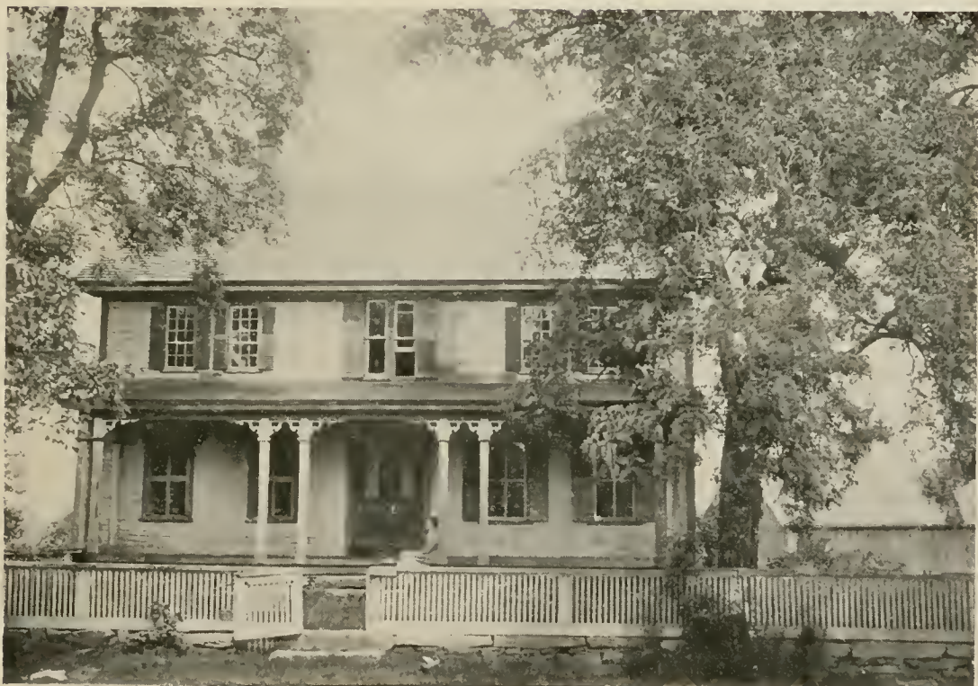
HOMESTEAD OF JOSHUA GRANT (1142, 30) AT NORTH STONINGTON
