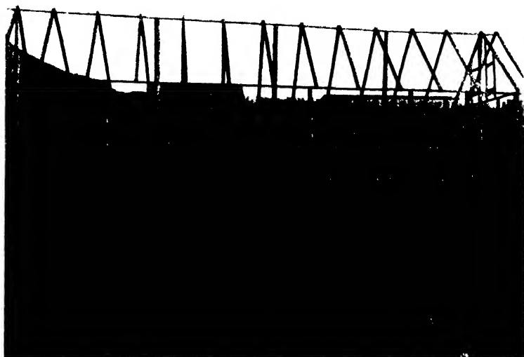
Photograph showing framework before thatching.
