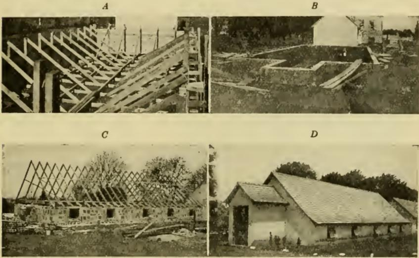
FIG. 156.—Four views showing construction of hollow-tile incubator cellar. A, Forms ready for pouring concrete foundation wall; B, forms removed; C, hollow-tile construction and manner of framing roof; D, completed cellar.
