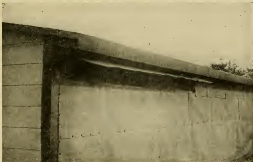
FIG. 67.—An efficient rear ventilator for summer use. It allows the air to enter the back of the house, and circulate between the sheathing and the roof, cooling the roosting quarters on summer nights. This is most valuable for shed-roofed houses that are covered with paper. Cornell University was the first Experiment Station to recommend back ventilation for the poultry house.
