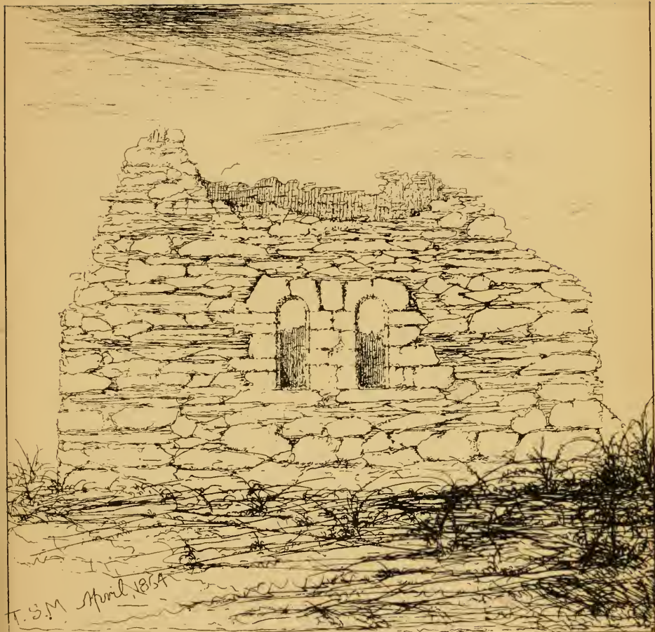
KILMORY-KNAP, EXTERIOR EAST END ELEVATION.
