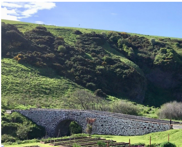
Bridge at Nethermill built in 1719
