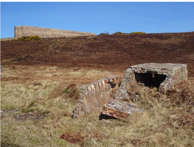
As I continued up the hill, I found a more intact structure. It was roofless, but the three-brick-thick walls had survived the best attempts of time, wind and vandals to knock them down.
