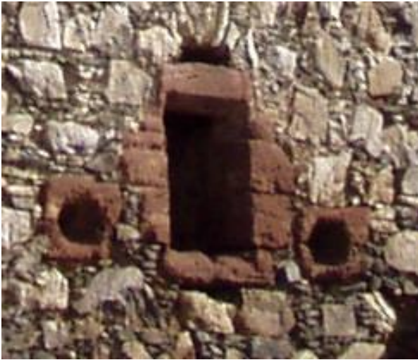
Gun ports on south wall. (S. Bruce).
