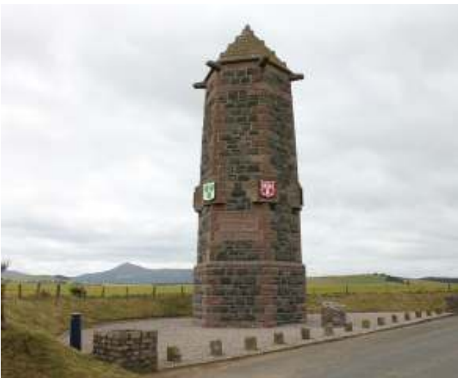
The Harlaw Monument with Panels attached and Bennachie in the background.
