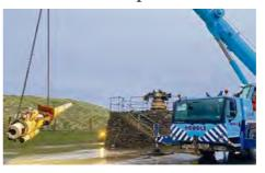
Orkney contractors have successfully eased 100-year old naval guns from their plinths at the Scapa Flow Museum. In a delicate operation barrels were disengaged from mounts and century-old screws removed - with no cutting required - as the guns were removed from their plinths and dismantled in preparation for storage or transport to await conservation work. The guns - which are two of only five First World War German naval guns surviving
