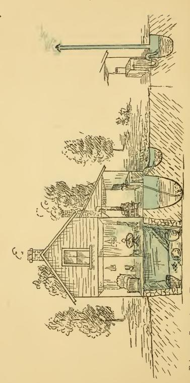
Poisonous Gases in our Houses. The blue shading shows the poisonous gases arising from decaying vegetables and badly constructed cesspool. Much of the sickness prevalent in the spring is due to these causes. A properly constructed cesspool is shown at the right. An S crook in the pipe prevents the return of gases, while the ventilating shaft carries them off.
