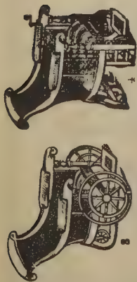
Nos. 3 & 4 are self-propelling Chairs, one mounted upon engine-cut cogwheels, the other with 24-inch rim wheels outside; either may be used by a child eight years of age with the greatest ease.
