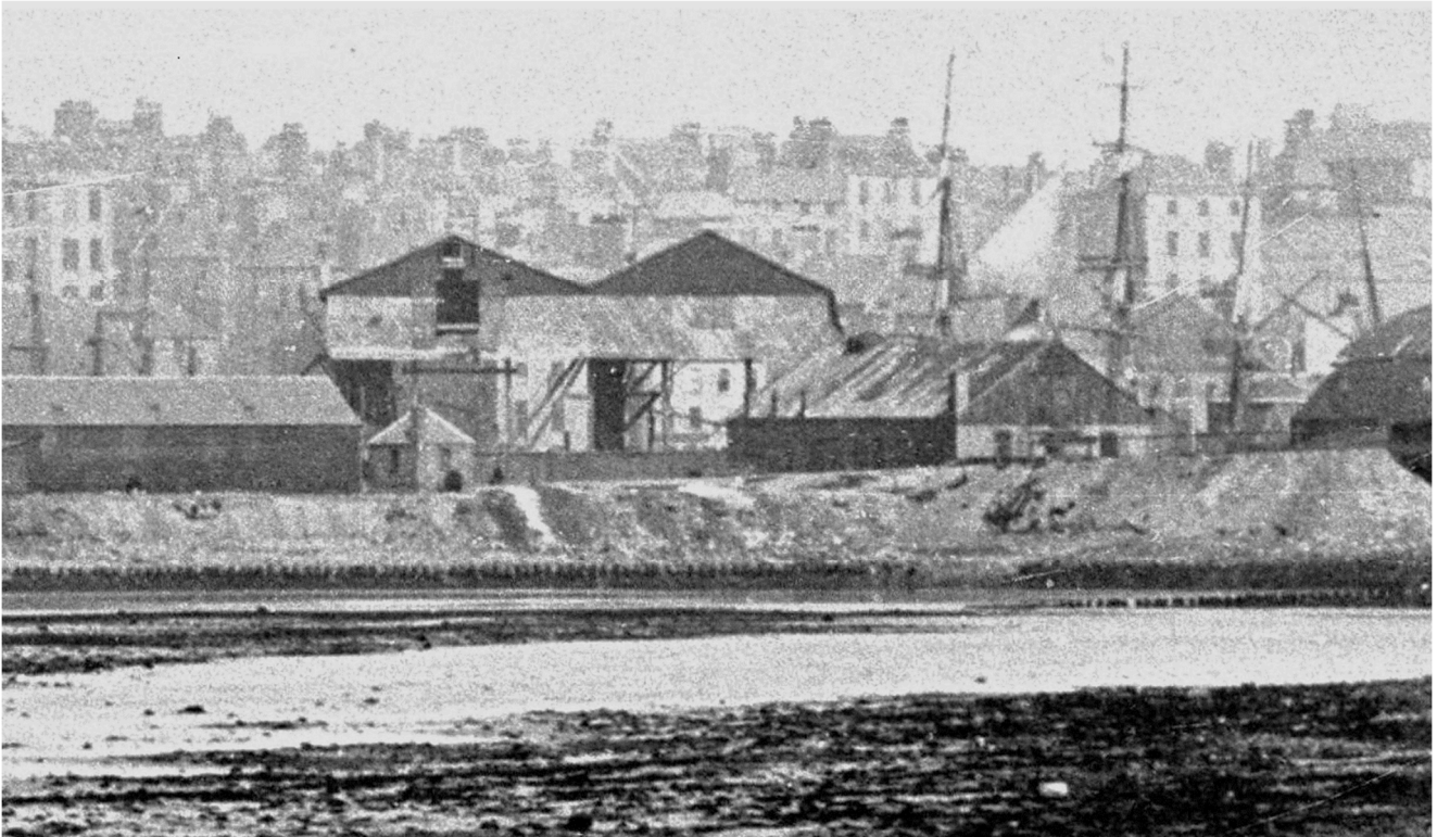
View of William Duthie Junior's building sheds, viewed from the south, 1869. (Photographer unknown).
